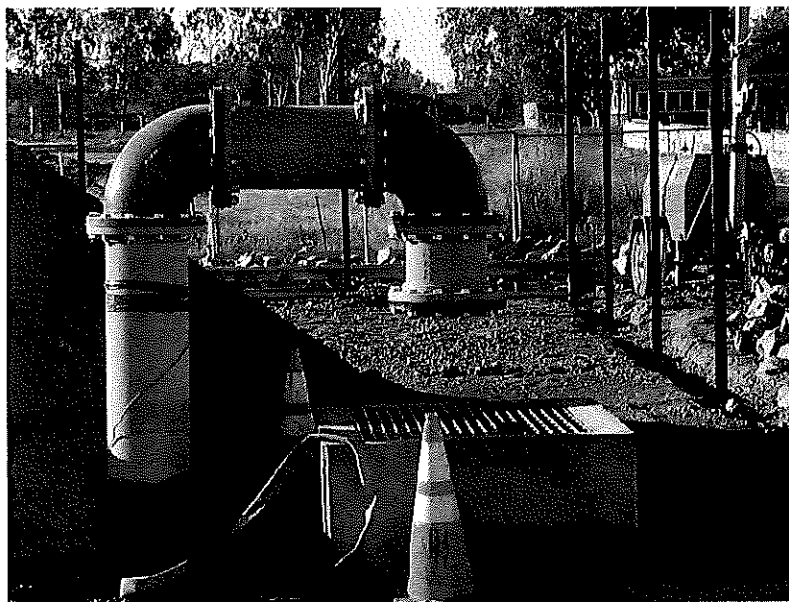
Well 16 pump to waste air gap structure
