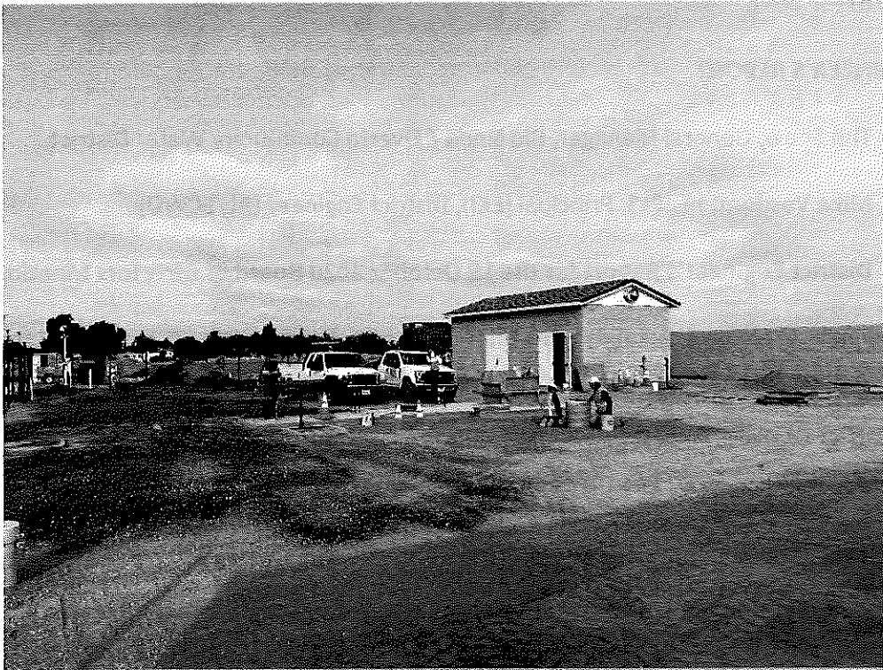
Well 16 site construction progress
