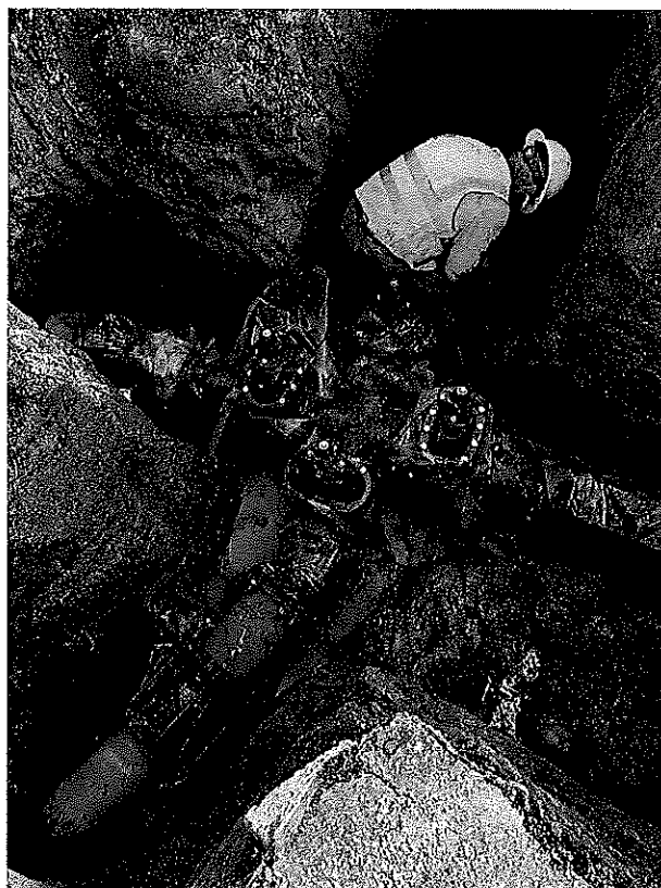
New cross and valve replacement
