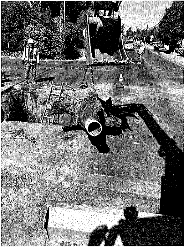
Existing valve cross @ Q Street
