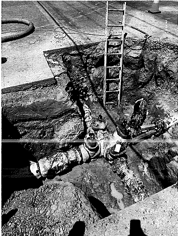
New valve cross @ Q Street
